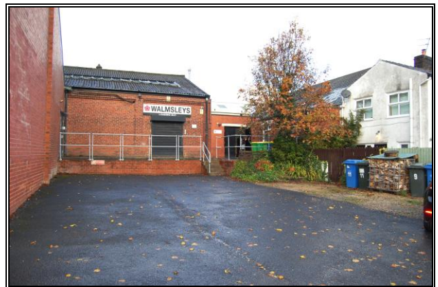
Rear Loading Bay
